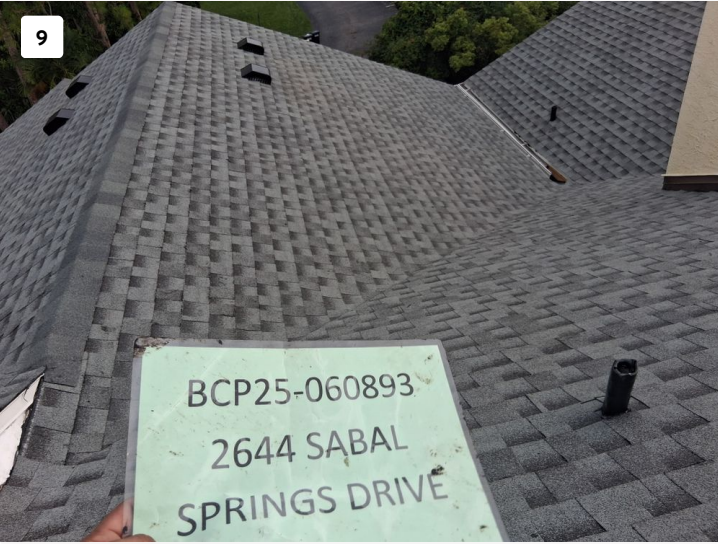
Project: WESTCHESTER SHORES - MASTER / 2407-5882872-01 Date: Jul 14, 2025, 6:34 PM Creator: Lucio Roofer
