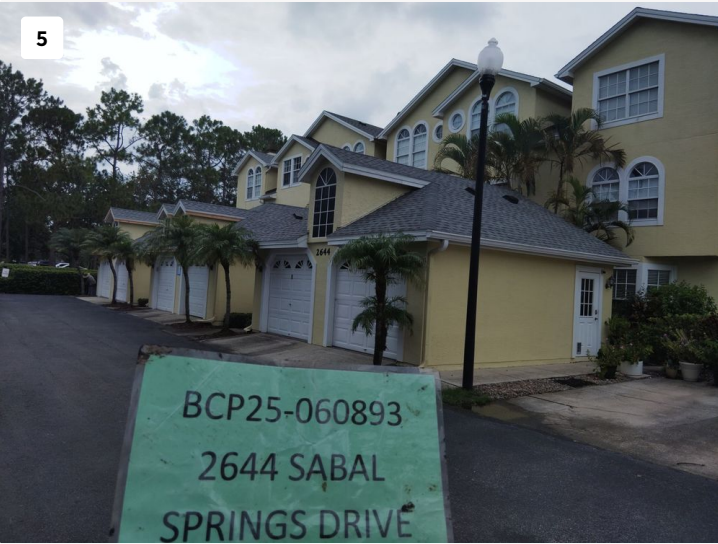
Project: WESTCHESTER SHORES - MASTER / 2407-5882872-01 Date: Jul 15, 2025, 6:46 PM Creator: Lucio Roofer
