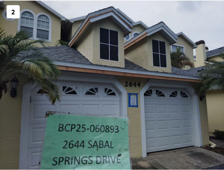
Project: WESTCHESTER SHORES - MASTER / 2407-5882872-01 Date: Jul 15, 2025, 6:38 PM Creator: Lucio Roofer
