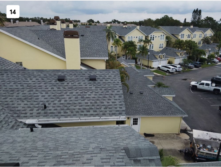
Project: WESTCHESTER SHORES - MASTER / 2407-5882872-01 Date: Jul 15, 2025, 2:48 PM Creator: Lucio Roofer
